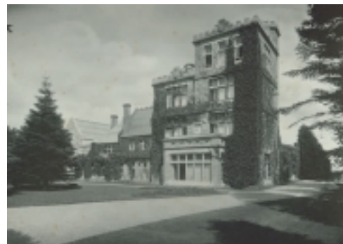
Shaw Royd House: an exterior view, which does not do justice to the magnificent gardens.
